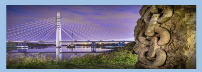
The new road bridge is a two-span cable-stayed bridge with an A-frame pylon rising to 105m (344ft) crossing the River Wear between Castletown on the north to Pallion on the south bank.
