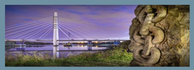
The new road bridge is a two-span cable-stayed bridge with an A-frame pylon rising to 105m (344ft) crossing the River Wear between Castletown on the north to Pallion on the south bank.
