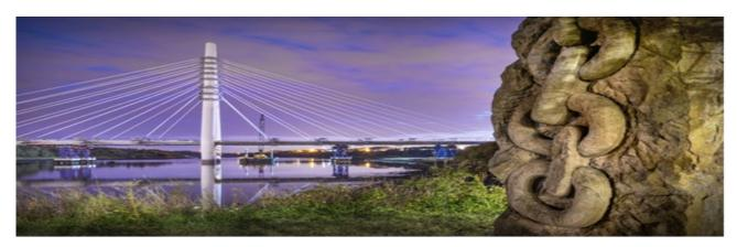
The new road bridge is a two-span cable-stayed bridge with an A-frame pylon rising to 105m (344ft) crossing the River Wear between Castletown on the north to Pallion on the south bank.
