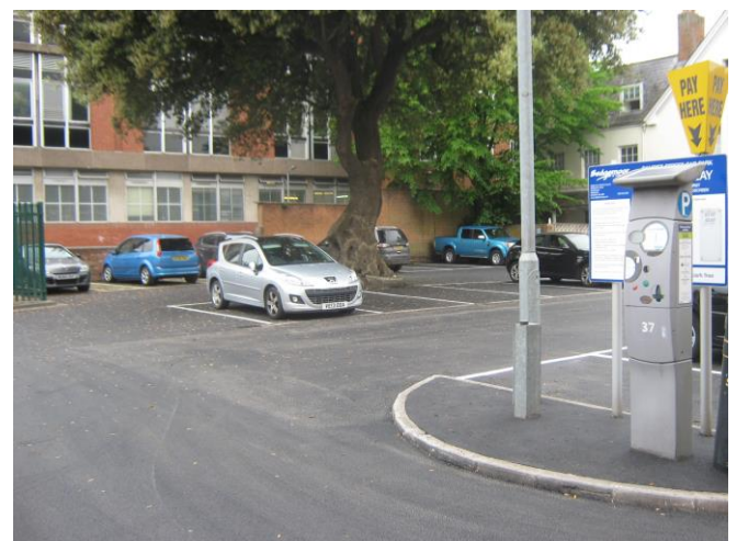
Dampiet Street car park, Bridgwater after resurfacing
