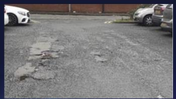
Sometimes patch repairs are not enough and a complete resurfacing of car parks is required. This means closing a car park for several days while a team comes in to remove the existing surface and prepare for resurfacing and then relining. We will always communicate such closures both on site and through our web pages, well in advance, to minimise the inconvenience to our customers.
